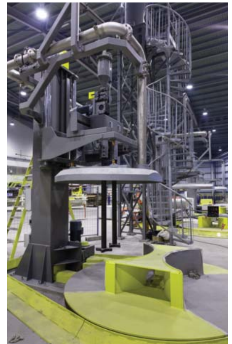
VHE Molten Metal Station during installation.
